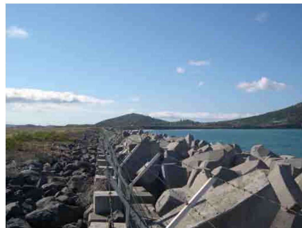
Figure 17 – Photo de blocs ACCROPODE™
