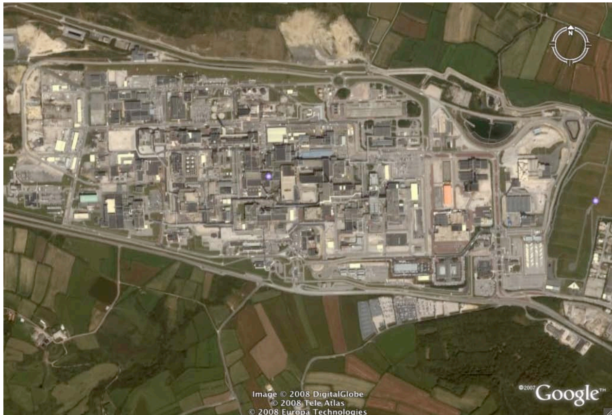
Figure 5. The reprocessing complex at La Hague. The site comprises the old UP2-400 plant and the operating plants UP2-800 and UP3 and their annex facilities (spent fuel storage, waste treatment).
