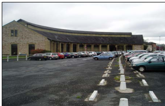
Parking personnel SNCF
