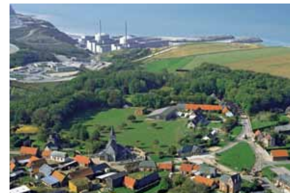
Le village et la centrale de Penly.
