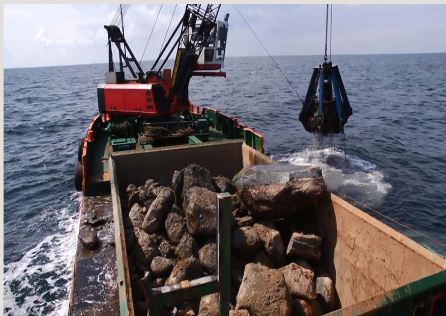
Chantier Dong Energy
